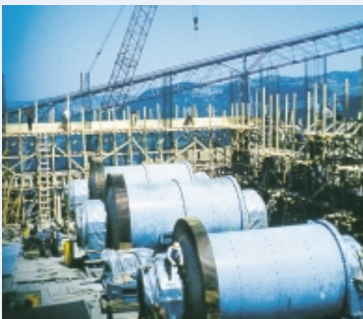
Delivery and installation supervision of 4 copper ore grinding mills, \varnothing 5.3 x 7.8 m.
